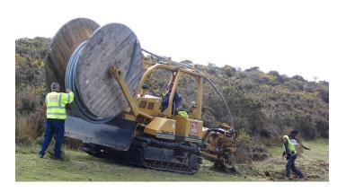
Work started on 13th April 2021 to lay a fibre optic cable across Gibbet Hill from Mary Tavy to West Blackdown. It took only a day to bury 1.85km of conduit pipe beneath the moor. Work to pull the new underground fibre cable through the conduit and to connect individual homes in West Blackdown will commence on 26<sup>th</sup> April.
